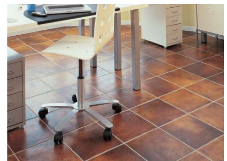
Underfloor heating with tiles
