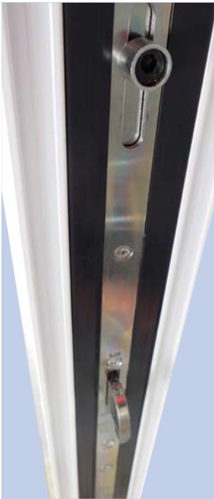
View of lower hook bolt and cam
